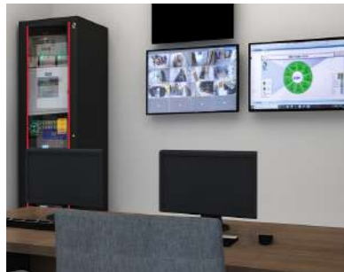
Data Center Monitoring Solutions
