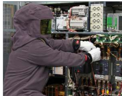
Service: • AMC • Mission Critical Facilities Management Services
